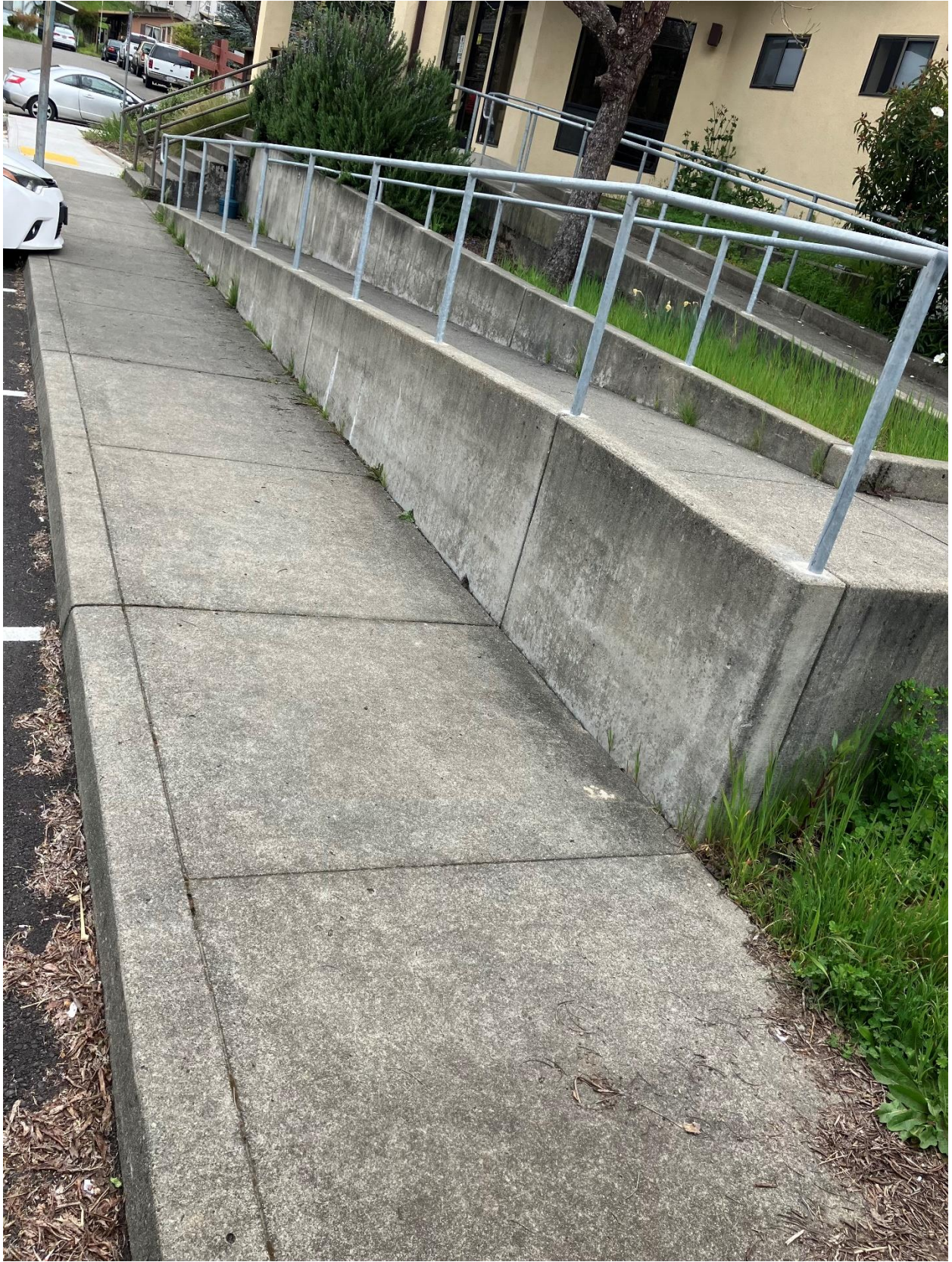
Redway site photo 3 of 3
