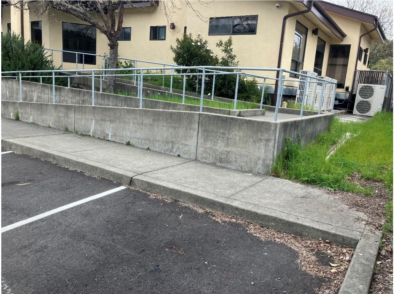
Redway site photo 2 of 3
