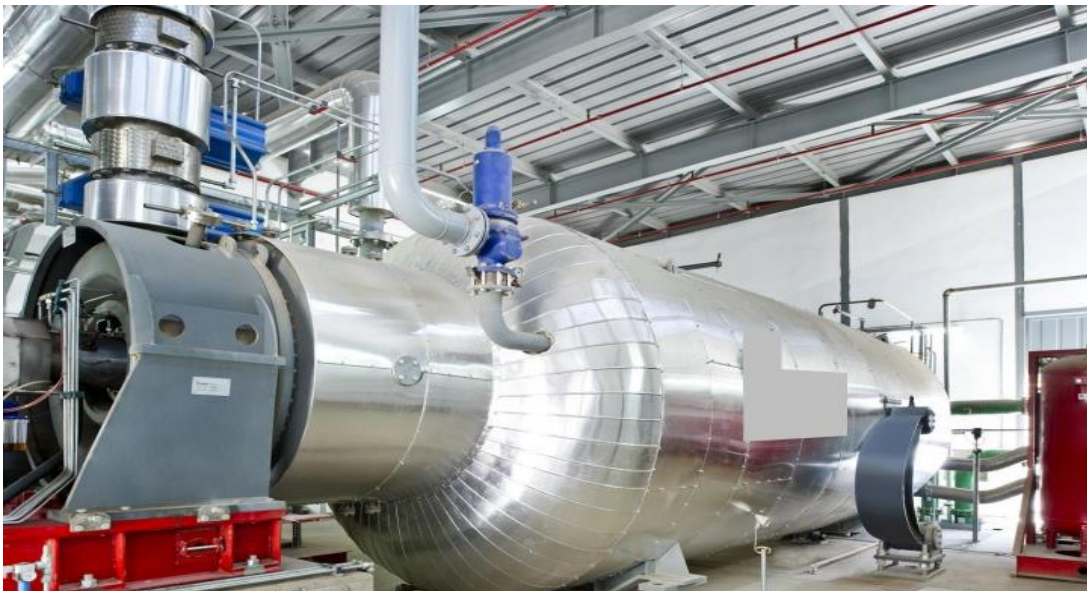
Figure 6. Modular scale, Organic Rankine Cycle (ORC) system (Turboden 2020)
