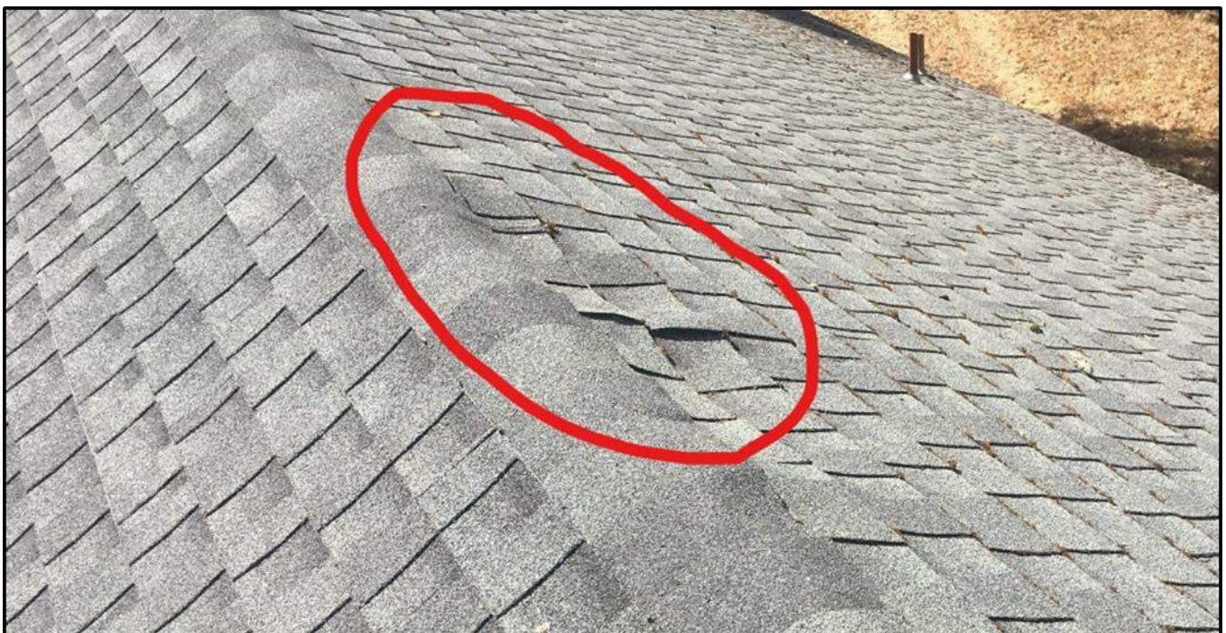
Figure 11 Potential roof damage on northwest face of the roof at Honeydew Elementary School.
