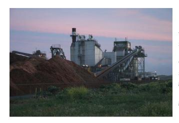
Fairhaven Power is located approximately five miles from Eureka, California, in Samoa, it started commercial operation in 1986. The plant generates power from burning woodwaste in a Riley inclined water-cooled stationary pinhole stoker boiler. The steam generated by the boiler powers an 18.75 (gross) MW Westinghouse steam turbine generator. The facility operated under a long-term Power Purchase Agreement with PG&F for most of its life. PG&F would not
