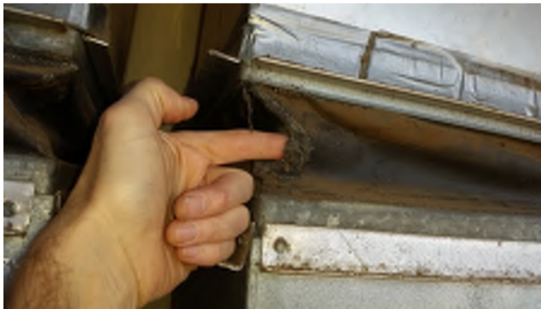
Figure 20. Large leaks in Wood Shop furnace supply plenum
