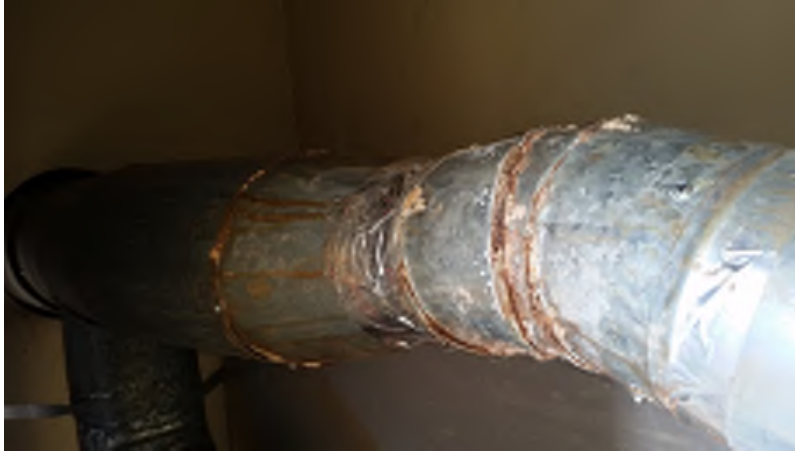
Figure 21. Corrosion of common shared flue in Wood Shop furnace closet
