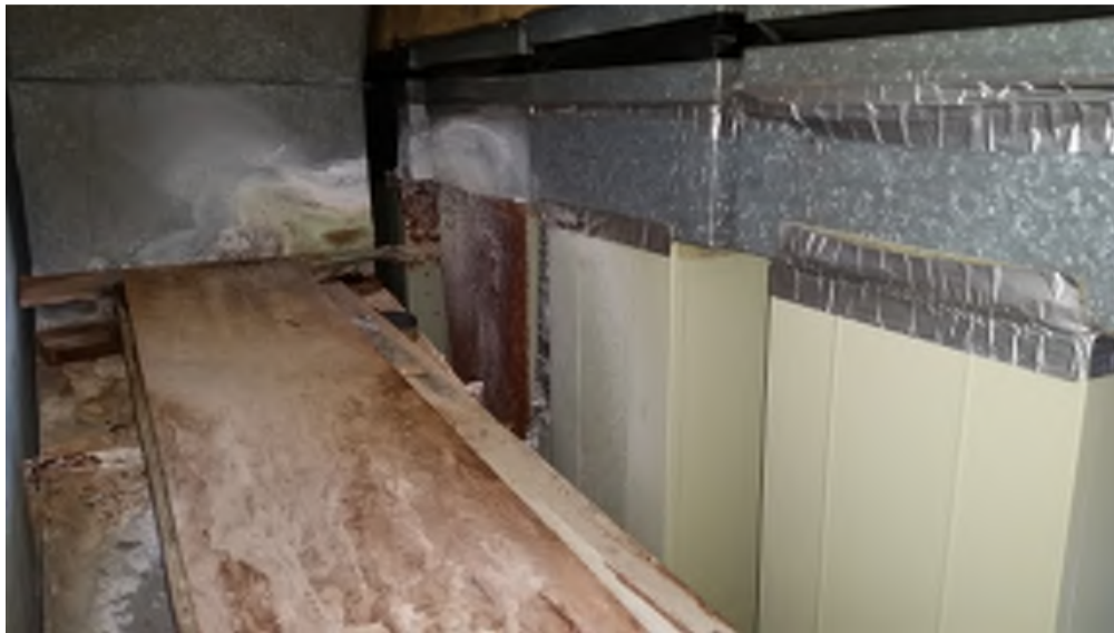
Figure 7. Shared return plenum behind Building A furnaces
