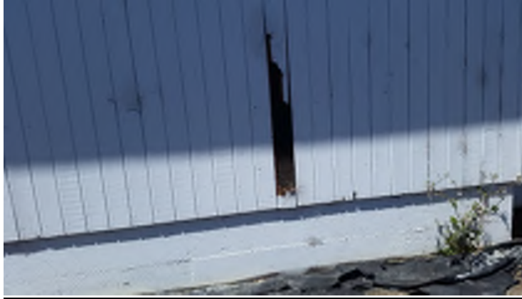
Figure 26. Moisture damage to siding of Music Building
