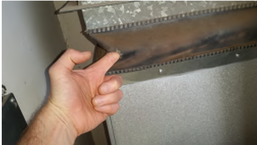
Figure 28. Leak in supply plenum of Ceramics Lab furnace
