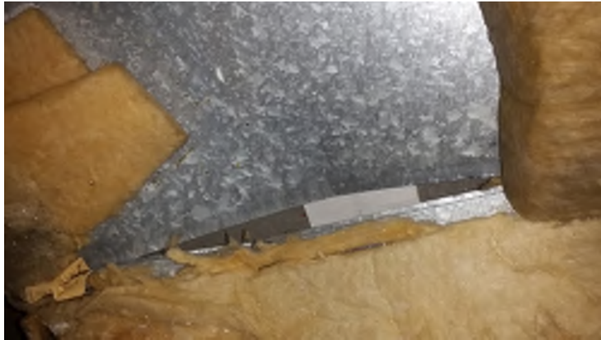
Figure 18. Collapsed duct with major leak above classroom F5
