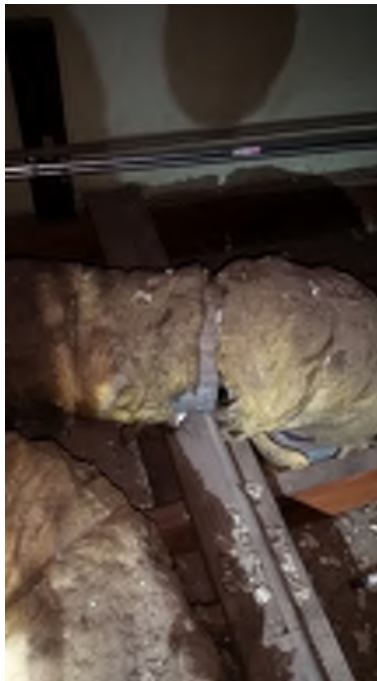
Figure 14. Severely compromised ducting in Auto Shop Classroom furnace
