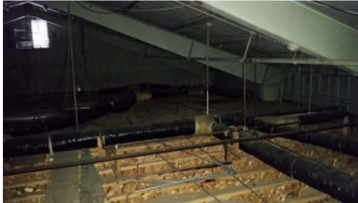
Figure 15. Long duct runs to a total of 10 registers from a single small HVAC system
