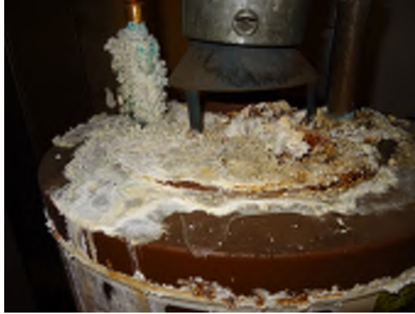
Figure 24. Failed water heater in Ag Building attic
