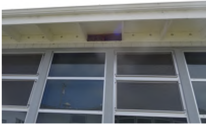
Figure 11. Building D missing eave block
