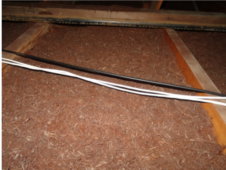
Figure 11. Photo depicting existing redwood bark insulation in Classroom and Administration Building attic.
