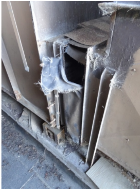
Figure 14. Image showing destroyed seal on Gym rooftop fan coil/air handler (AHU).
