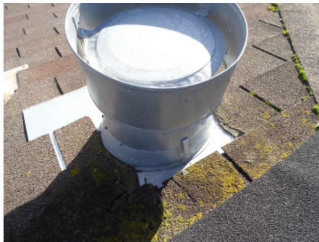
Figure 3. Image illustrating damaged roofing material around roof penetration.
