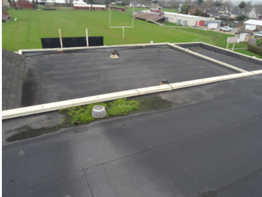
Figure 13. High School Gymnasium roof detailing configuration and maintenance issue around drainage scupper.
