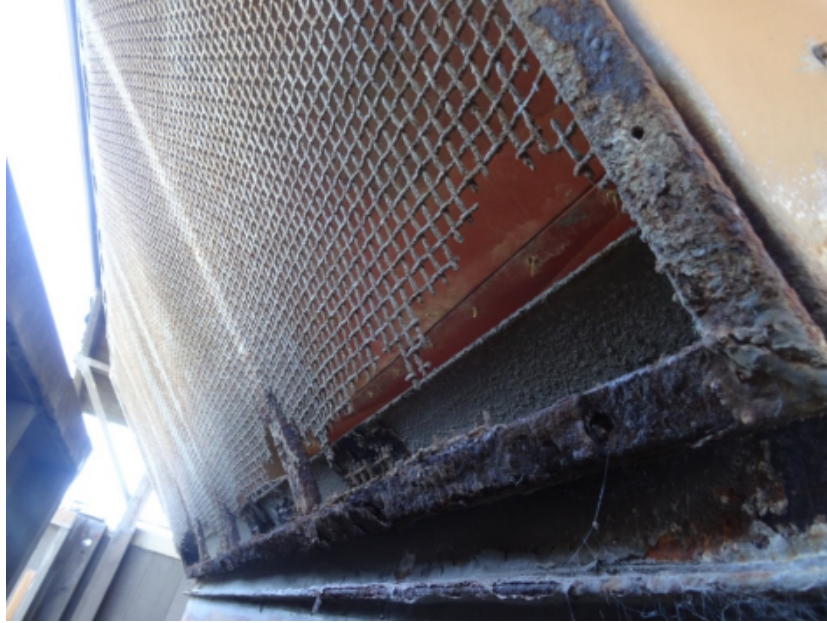
Figure 15. Image showing significantly corroded high school gym roof top AHU outside air intake screen and cabinet.
