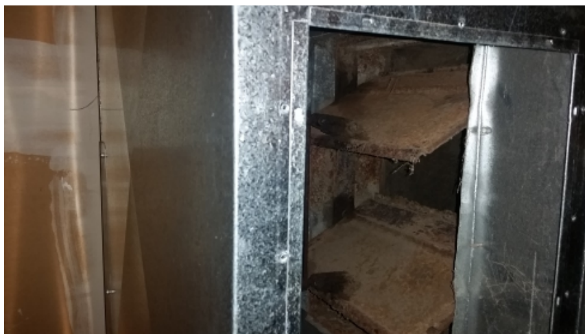
Figure 8. Image showing elementary school gym OSA damper in fully open position.
