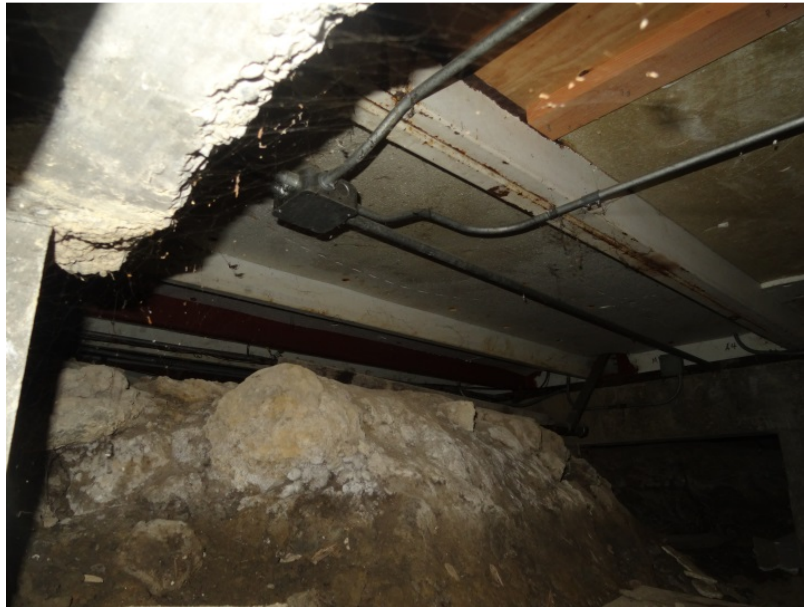
Figure 5. Photo showing uninsulated gym floor, excavated perimeter and limited crawlspace access.
