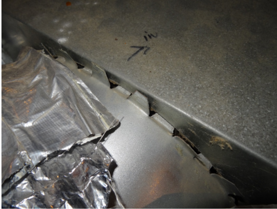
Figure 7. Image detailing duct leakage location at return air plenum/flex duct connection point.
