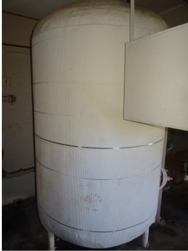
Figure 16. Ferndale High School Gym 400-gallon DHW storage tank.
