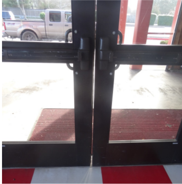
Figure 12. Image illustrating missing weatherstripping on Gym exterior door.
