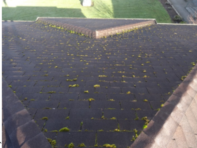
Figure 2. Image showing north side portion of roof showing moss growth, lifted asphalt shingle corners and original redwood gutters.
