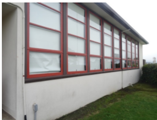
Figure 10. Image showing large facade of north facing single paned glazing.
