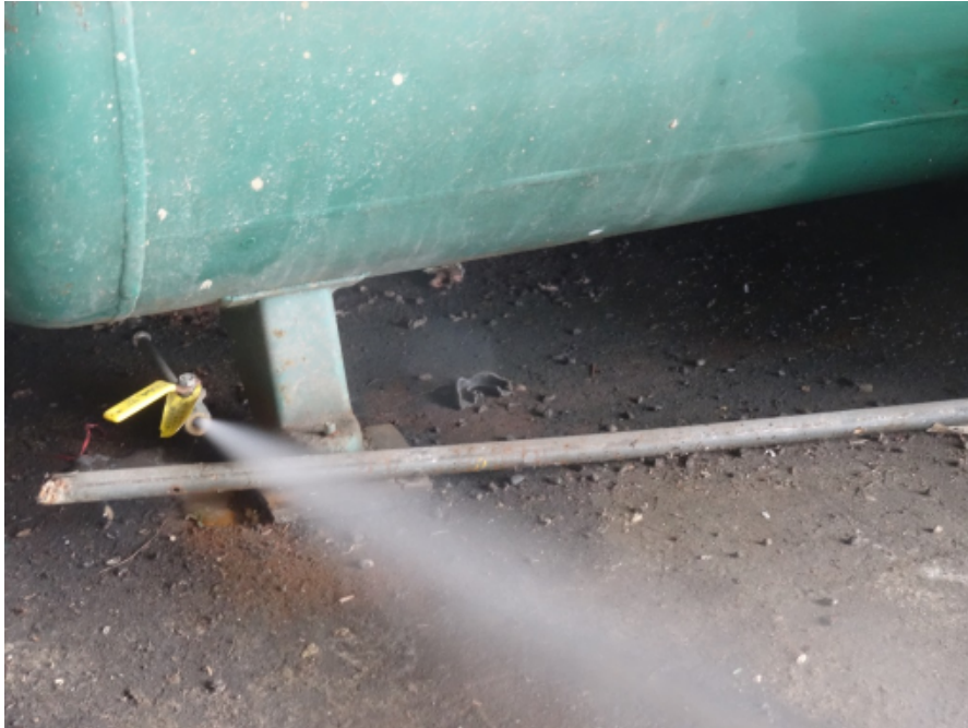
Figure 17. Image showing liquid condensate in Shop Class compressor purge stream.
