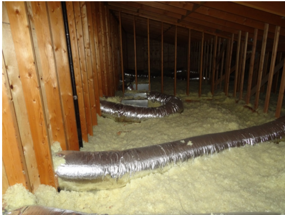
Figure 6. Image showing large amounts of flexible ducting used in Annex HVAC systems.
